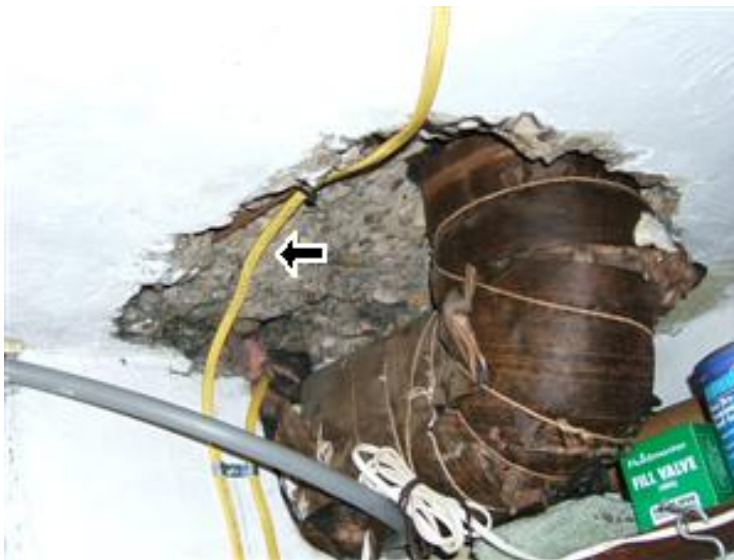
4.5 WALLS / CEILINGS Picture 1
