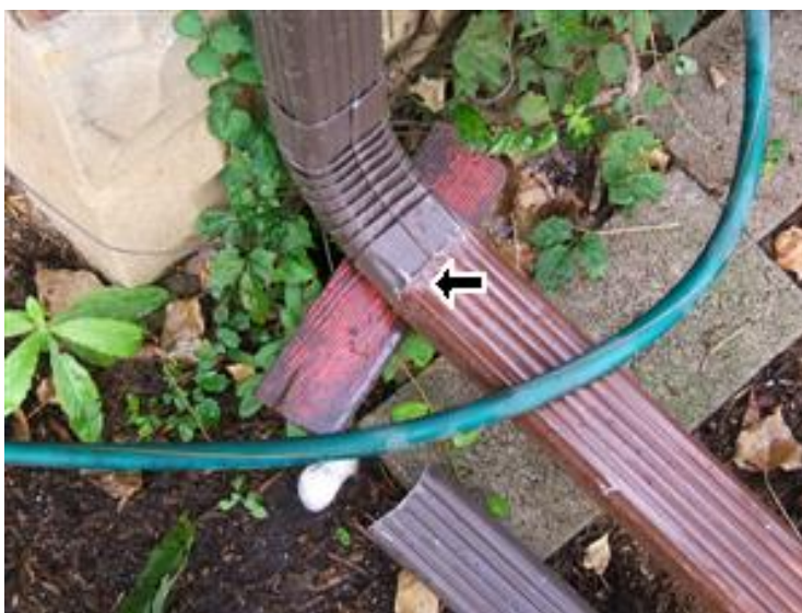
1.8 DOWNSPOUTS / ROOF DRAINS Picture 1
