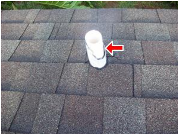
1.4 PLUMBING STACKS Picture 2
