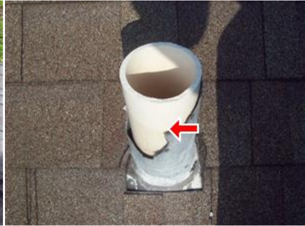
1.4 PLUMBING STACKS Picture 1
