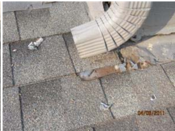
2.7 GUTTERS / DOWNSPOUTS / ROOF DRAINS Picture 1
