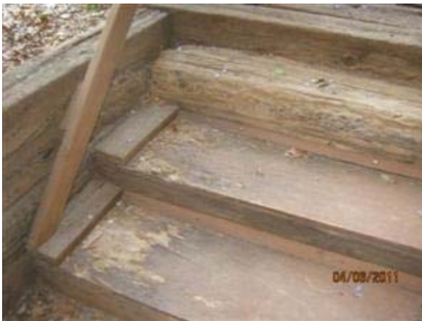
3.5 STAIRS / STOOPS Picture 1
