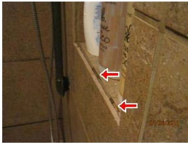
9.13 Master Bathroom WALL TILE / TUB SURROUND Picture 1
