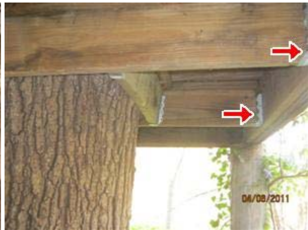
3.6 PORCH(ES) / DECK(S) Picture 1
