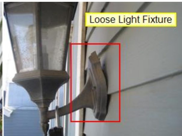
2.5 ELECTRIC / GFCI Picture 1
