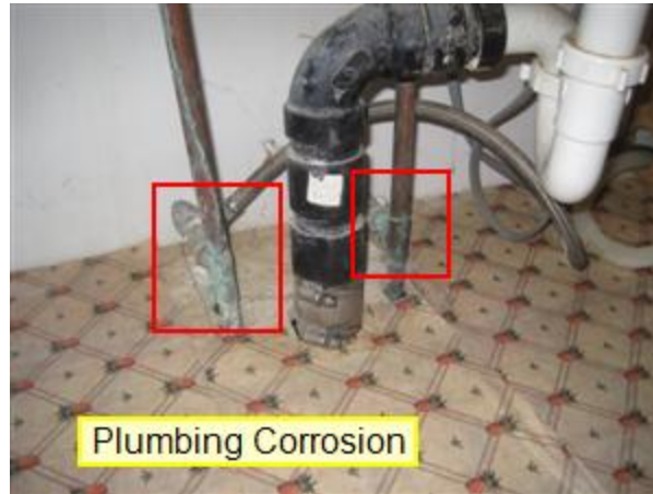
7.0 PLUMBING / SINK Picture 1
