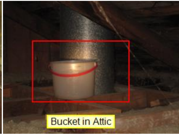
5.1 ROOF DECK / SHEATHING Picture 1
