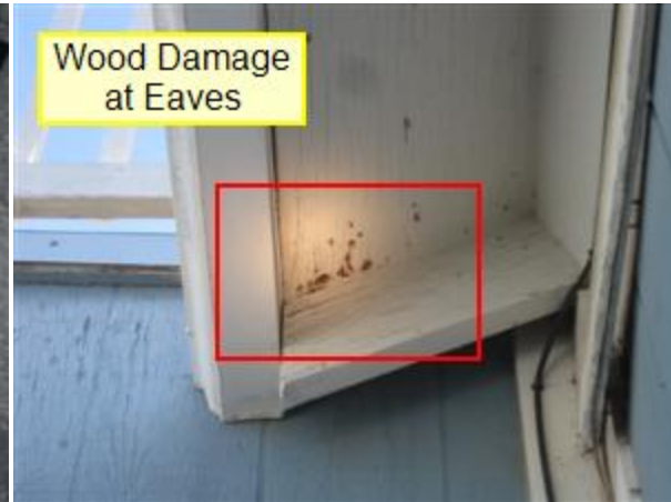
1.7 FASCIA / SOFFITS Picture 1
