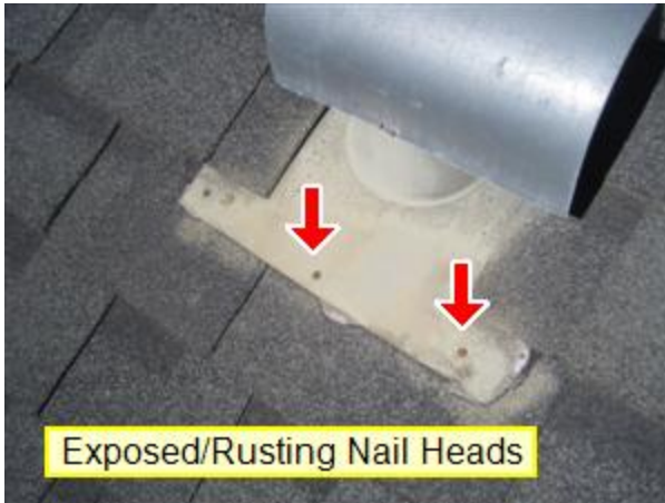
1.2 EXPOSED FLASHING Picture 1
