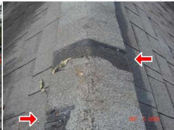
1.0 ROOF COVERING Picture 2
