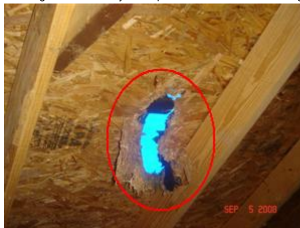
5.1 ROOF DECK / SHEATHING Picture 1
