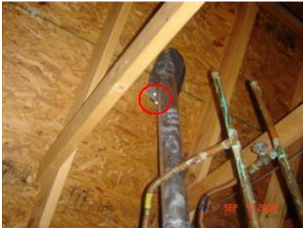
1.1 EXPOSED FLASHING Picture 1
