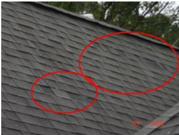
1.0 ROOF COVERING Picture 1
