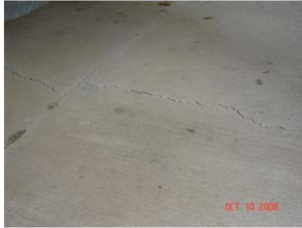
4.2 FLOOR SLAB Picture 1
