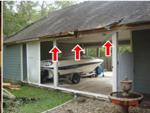
1.6 FASCIA / SOFFITS Picture 1
