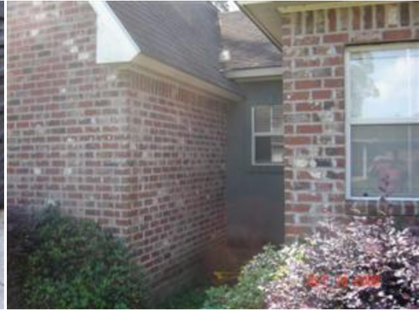
3.3 GROUND SLOPE AT FOUNDATION Picture 1
