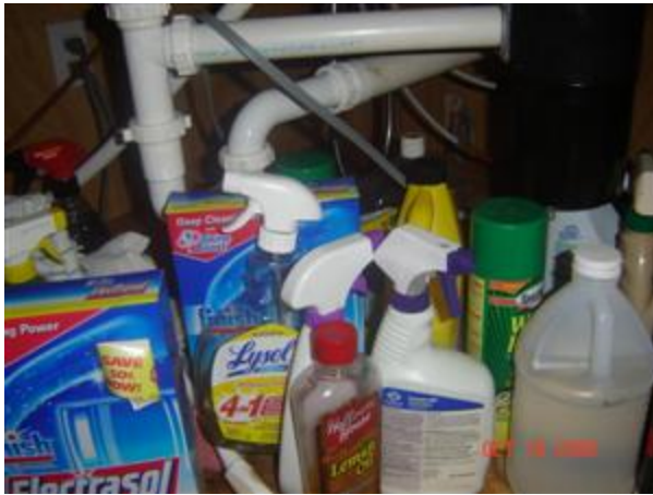
7.0 PLUMBING / SINK Picture 1
