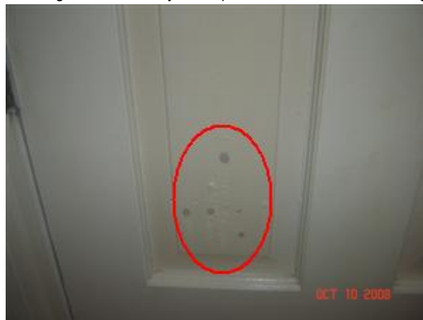
2.2 ENTRY DOORS Picture 1
