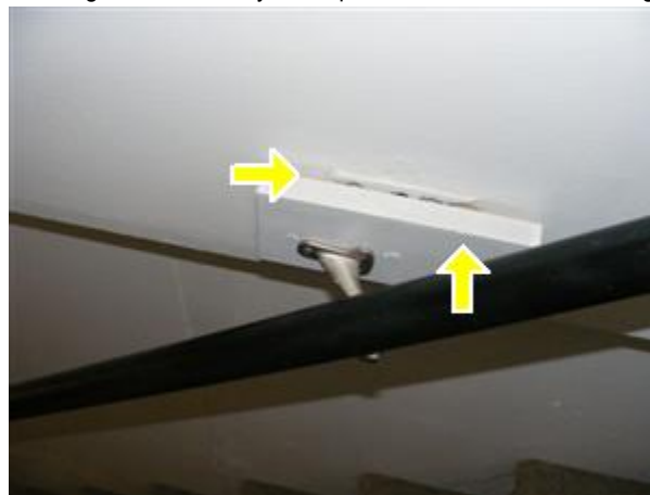
9.0 STAIRS / RAILINGS Picture 1
