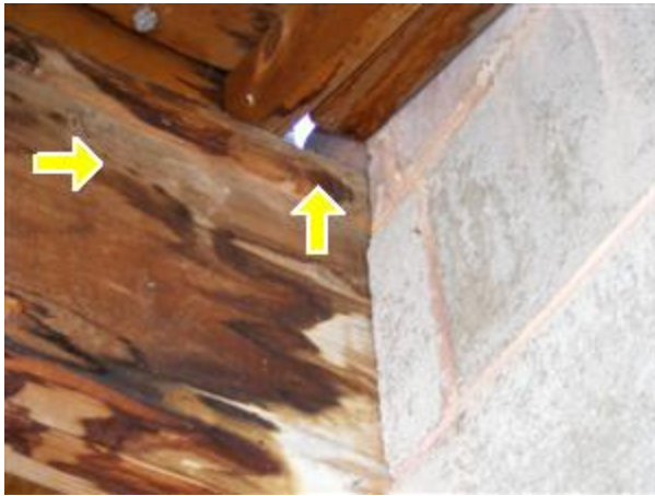
4.1 EXPOSED FRAMING Picture 1
