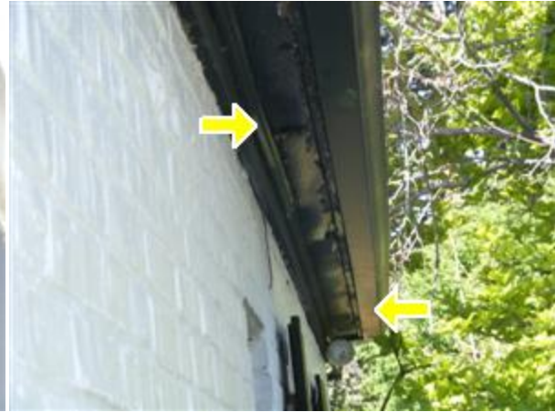
1.2 FASCIA / SOFFITS Picture 2
