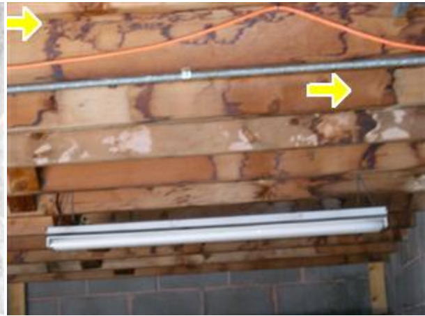
4.1 EXPOSED FRAMING Picture 2
