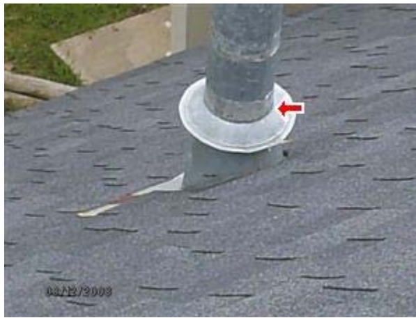
2.3 EXPOSED FLASHING Picture 3
